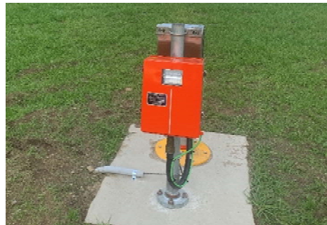
Figure 2-6: REIL During Construction
