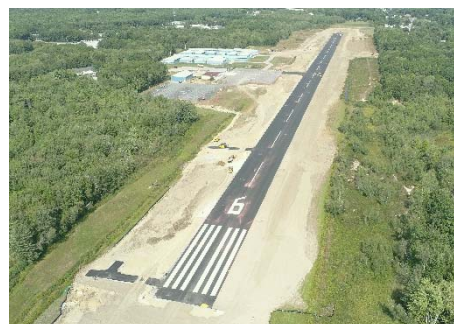
Figure 2-2: Runway 06-24 During Construction
