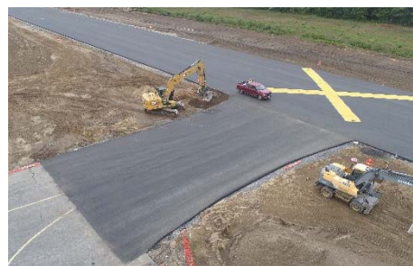
Figure 2-4: Taxiway During Construction
